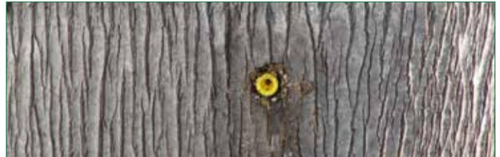
Plug slightly deeper than flush (1/16").
